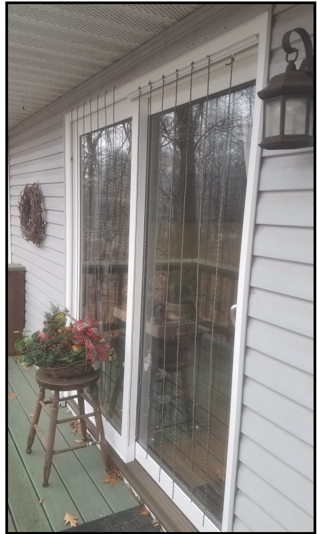
The new sliding glass door is now protected.
